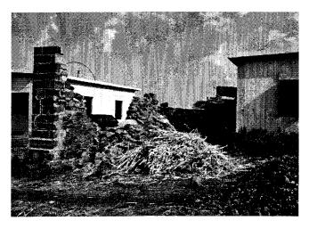
Fig. 8. Newly built wall that collapsed after only 2 monsoon seasons, new Sirsal, 1996. Photo courtesy of Rajendra Desai.
